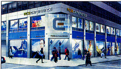
ICS Builders is constructing the new $1.7 million, 14,000-square-foot RCS Computer Experience store at 575 Madison Ave. in Manhattan.
