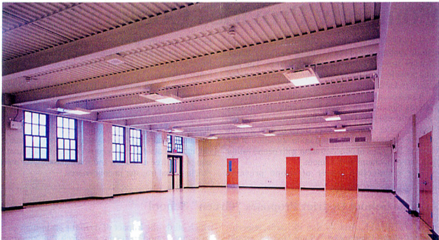
To address a shortage of classroom space, builders constructed a new floor horizontally across the height of the school's gym.
